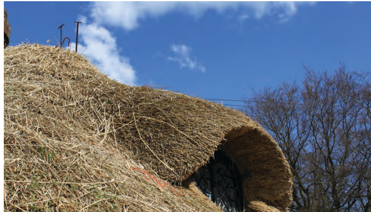
Above: Window detail, showing the treatment and overhang of the thatch. Top left is the new ridge being applied, and green shoots can be seen emerging from the surface.
