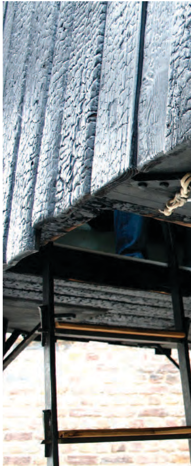
A detail of Fujimori's use of charred cedar for a small Tea House for the V&A in London
