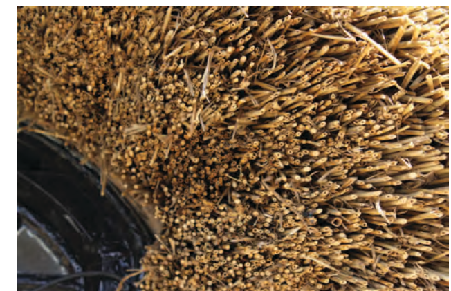
Above: Thatched window detail showing cut ends of longstraw. Photograph taken during a visit to observe a thatcher at work in Kent
