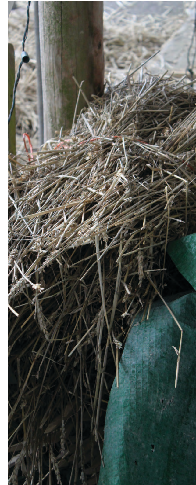
Above: Discarded straw to backfill the new thatch
