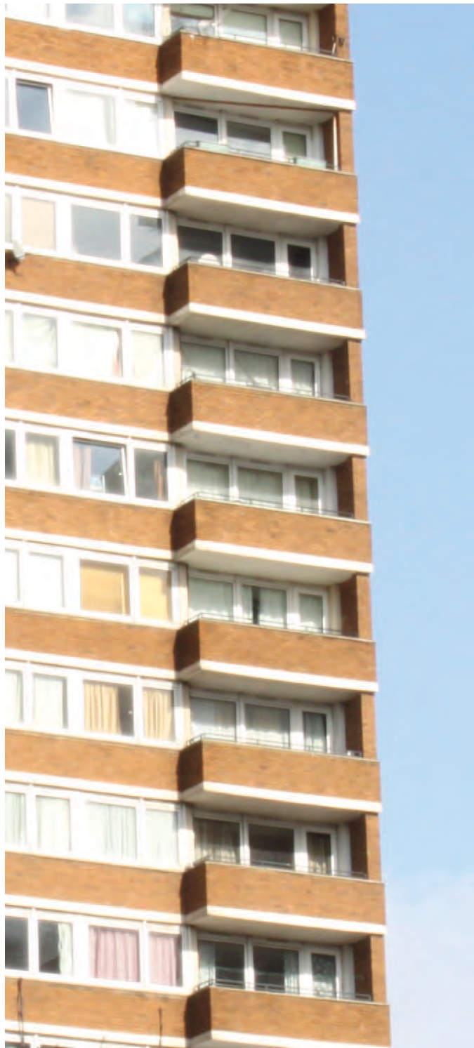
Elevation detail showing exposed slab edges
