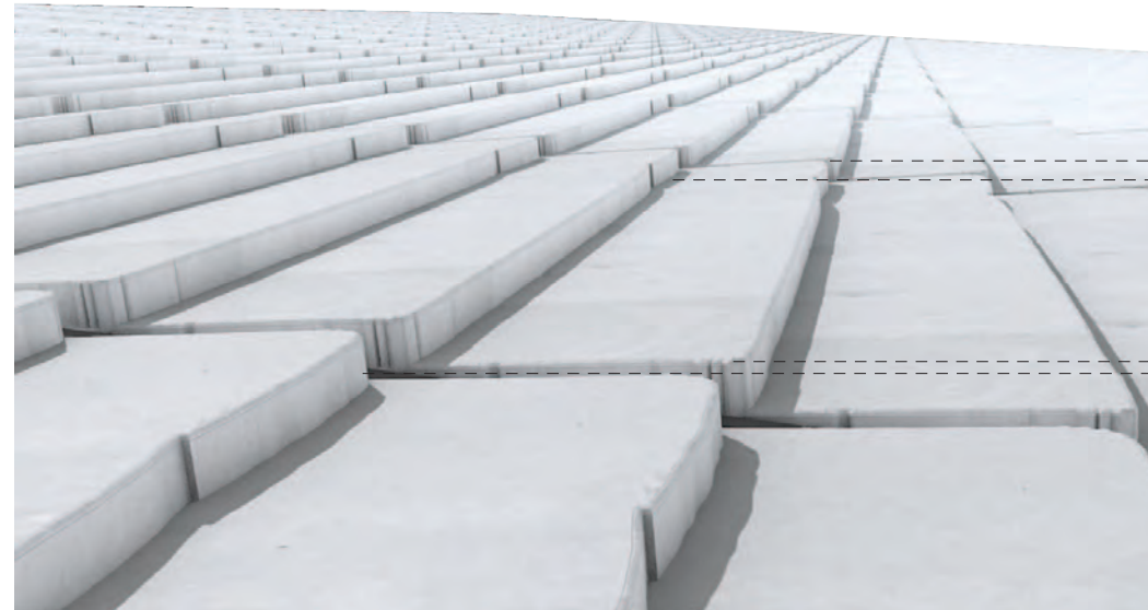
Roof detail. Lapped panels thickness 8 - 60mm (front to rear)
